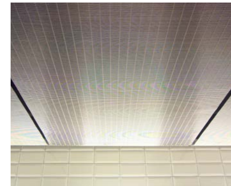
▲ Artos sigma 6: rigid in one direction, flexible in the other, and ideal for any facade
